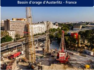
This water storage basin, of 50 metres in diameter and more than 30 metres deep, will store over 50,000 cubic metres of water. This project is an important investment of the Parisian city to control and manage the wastewater that currently is discharged into the Seine.
